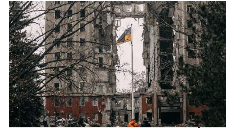
Destroyed city council building in Mykolaiv
